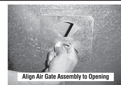
Figure 12 - Position Air Gate
